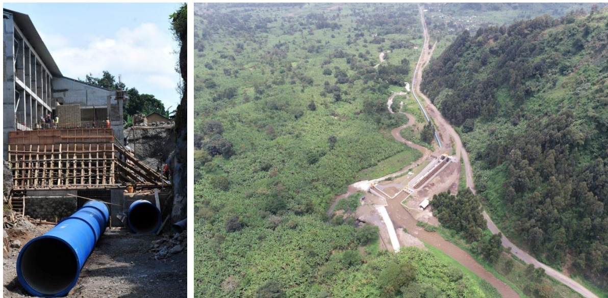
Fig.2. (Left) The two 4.5 km ductile iron penstocks of the Rwanguba scheme during construction, (Right) aerial view of the penstock in operation
