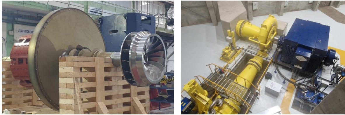
Fig.1. (Left) Francis turbine runner, generator rotor, and flywheel before assembly at Rwanguba, (Right) View of the installed Francis turbine-generator unit at Rwanguba
